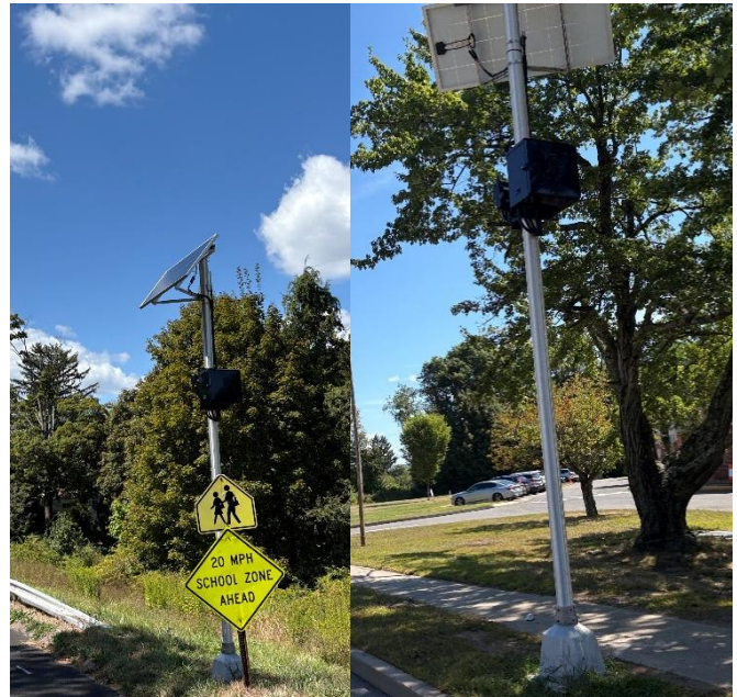
Signage and ATESD cameras located in Middletown
