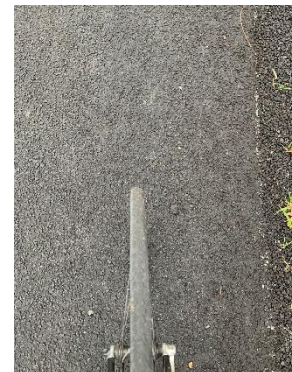
Photo 1: A chip seal surface with the new treatment.
