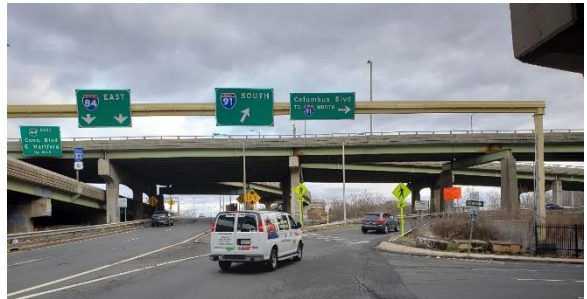
Photo 5: Bulkeley Bridge Marked Crosswalk
