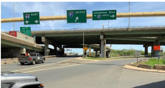
Photo 4: Bulkeley Bridge Unmarked Ped Crossing
